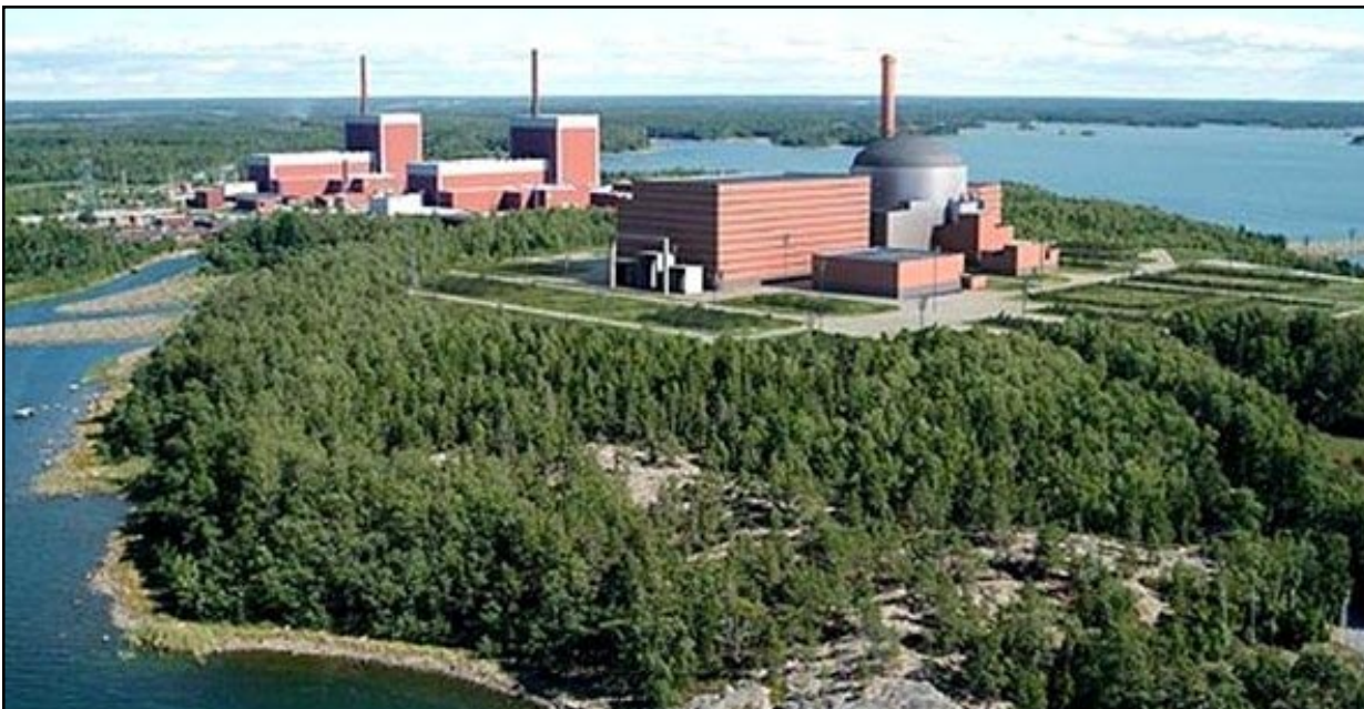
Finland's Olkiluoto nuclear power plant.
